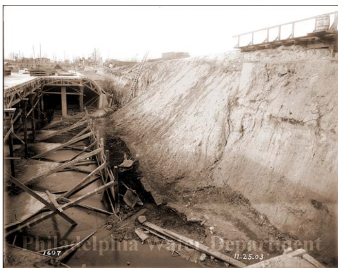
Torresdale Water Plant under construction in 1903
