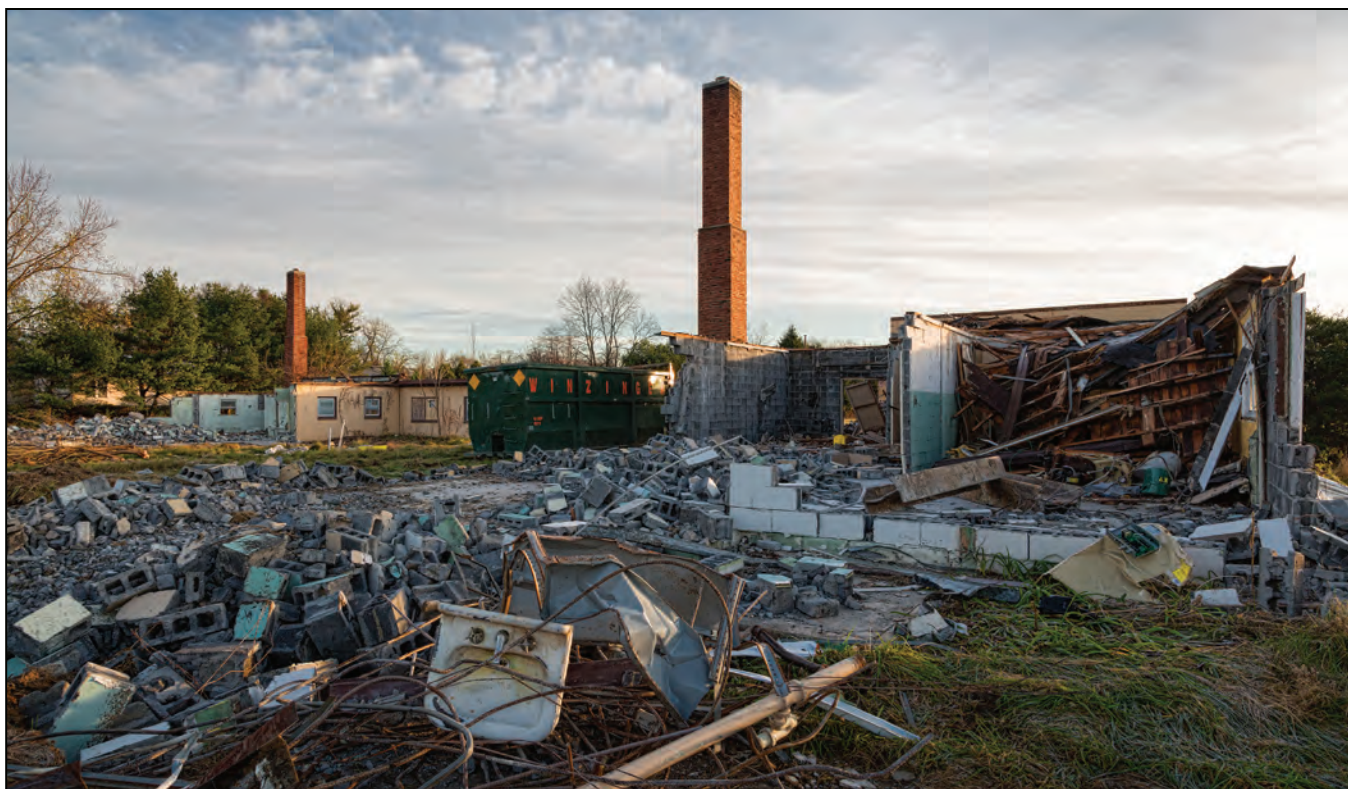
Demolition of radar site 2015. Photograph courtesy of Richard Lewis.
