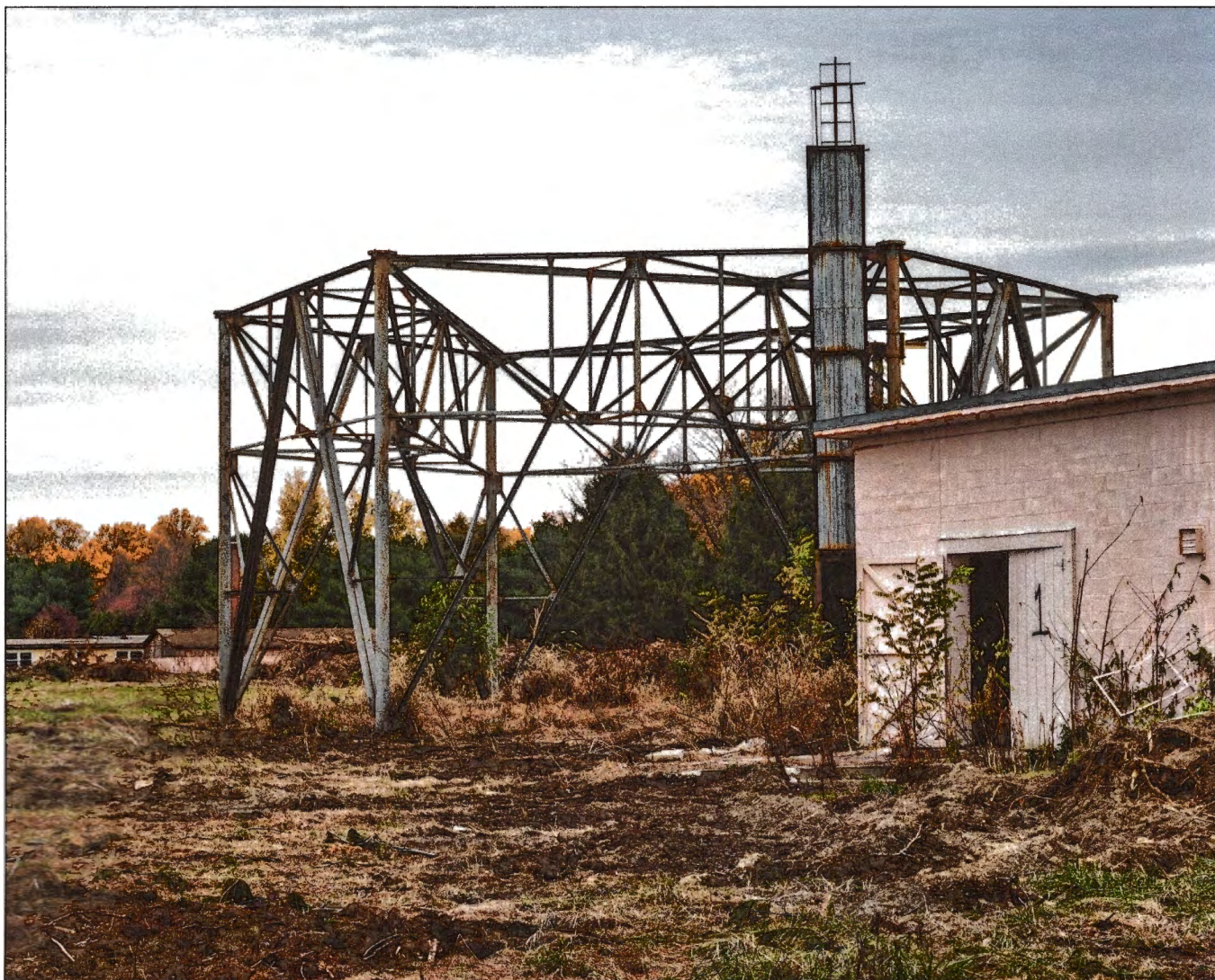
As seen in 2015 just before being dismantled to allow a housing development, this steel structure in Lumberton was the platform for a high-powered Nike Missile radar system. The actual antenna was mounted atop the structure, allowing it to scan out into the Atlantic, watching for incoming bombers; it would have been protected from weather by a fabric golf-ball-appearing radome. The adjacent building housed electronic equipment; other support buildings are in the distance. Photograph courtesy of Richard Lewis.
