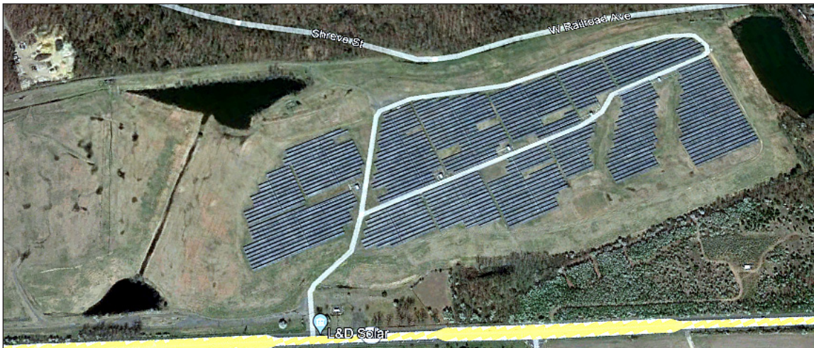
Partial view, Mt. Holly Landfill
