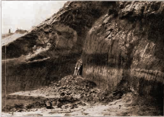
Northwest corner of recent opening of William Hoffman's Pit at Birmingham, Burlington County, N. J. Showing efflorescence and stratification of the greensand and creep along the face of the old bank, indicated by the contortion of sand-filled crevices.
