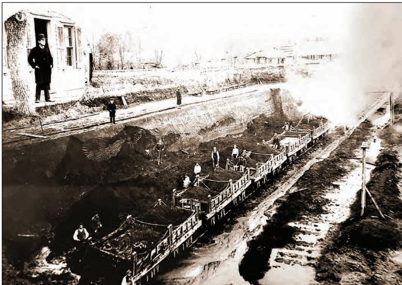
Marl pit at Sewell, c. 1888, later to become the Inversand Company operation. Note that as workers dug out the marl at the edge of the pit, the tracks would be repositioned to place them closer to the walls of the expanded dig area, facilitating manually loading the marl cars. 119
